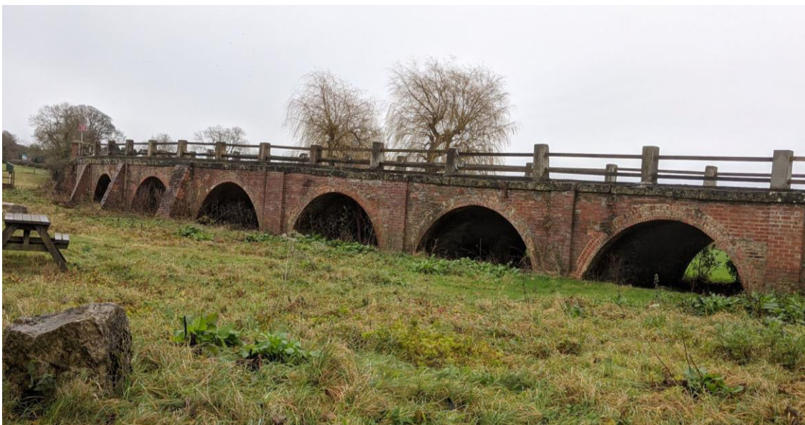
Figure 1: The 18C brick flood arches of the West approach with the 20C concrete posts and timber rails to the upstands, built in a curved line.
