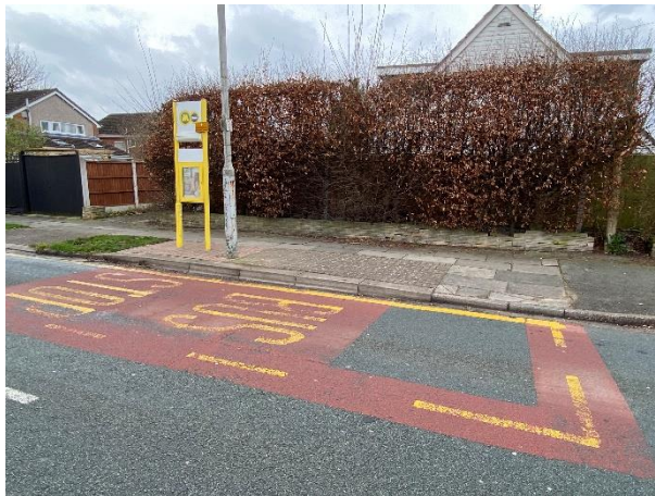
Figure 4.4 – Northbound Bus Stop (Brookhurst Avenue)
