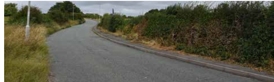
Narrow pavement running on the northern side of Gills Lane
