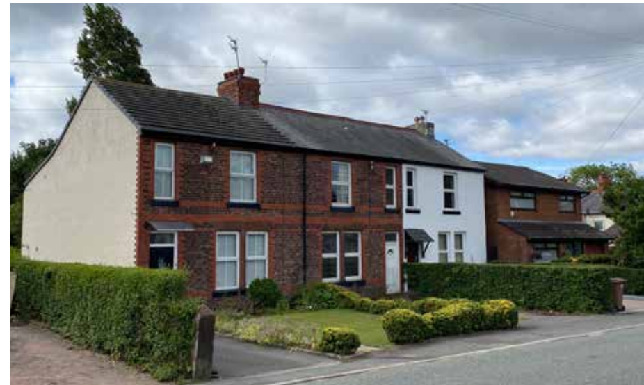
Red brick properties with large front gardens incorporating parking, Gills Lane
