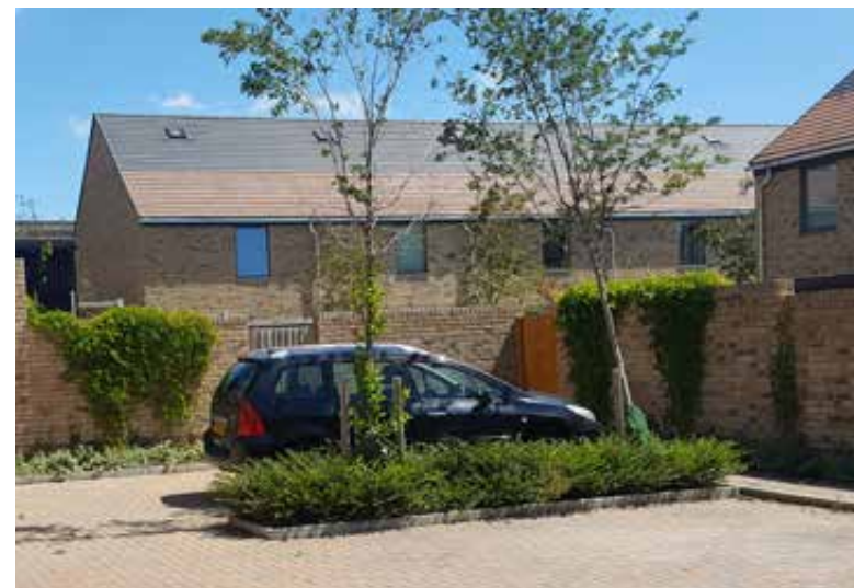
Rear parking court, Abode at Great Kneighton, Cambridge
