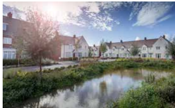
Homes overlooking open space
