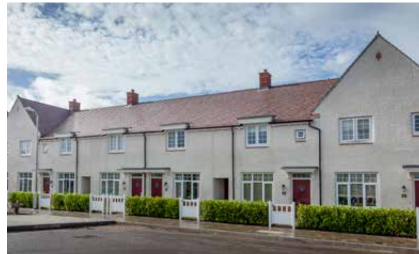
Terraced housing with hedged front gardens, Newport
