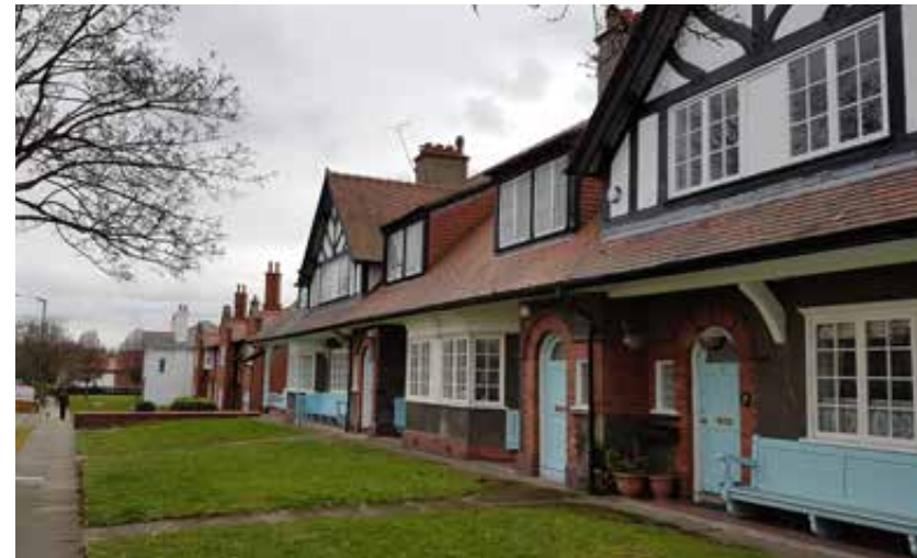
Terraced housing, Port Sunlight
