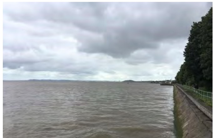
Eastham Ferry Looking South
