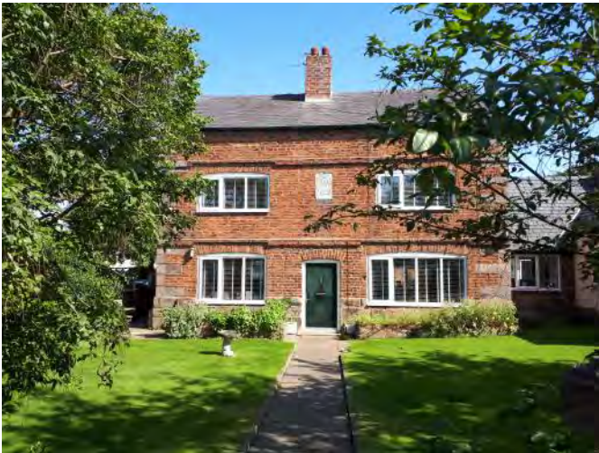
Grade II listed Poplar Farmhouse, Saughall Massie
