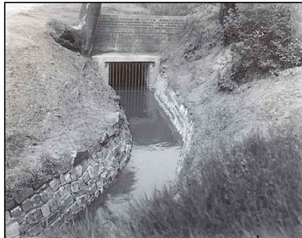
Fig 7. Stream with culvert and reinforced banks, photographed in 1927
