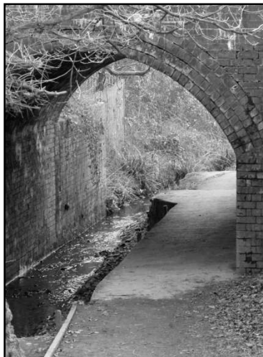
Fig 6. 'Echo Bridge' under the old Midland Railway line
