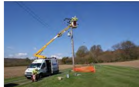
Removing overhead cables
