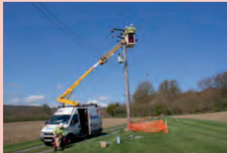
Photo: removing overhead cables
