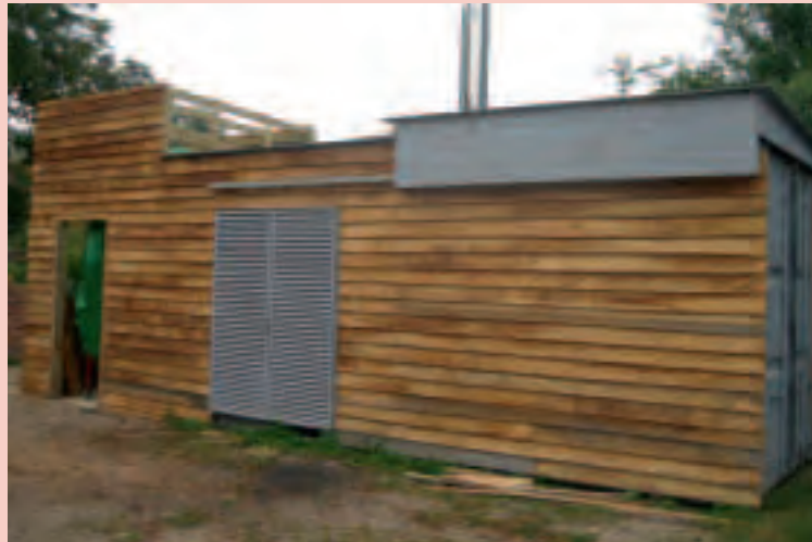
Photo: oak clad boiler housing
