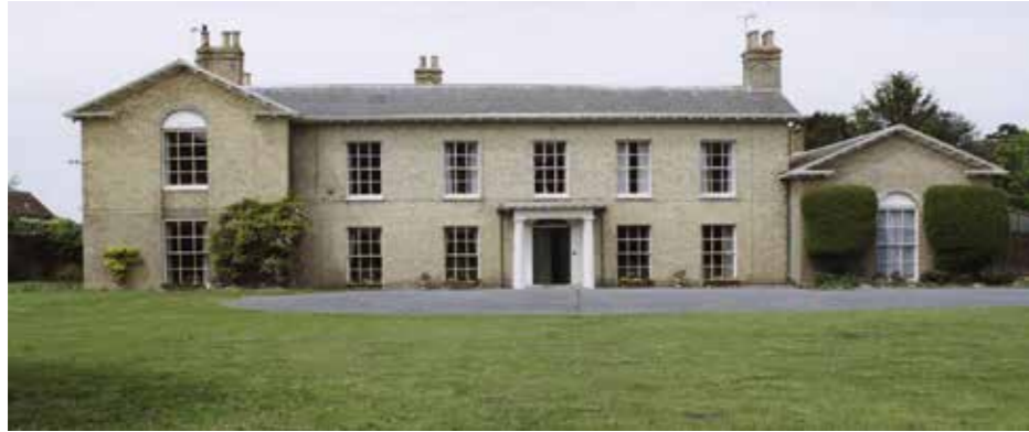
Figure 5.77 The principal east elevation of Rodmersham House
