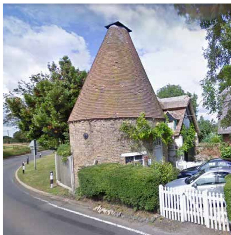
Figure 5.43 The Former Oast viewed from Tunstall Road
