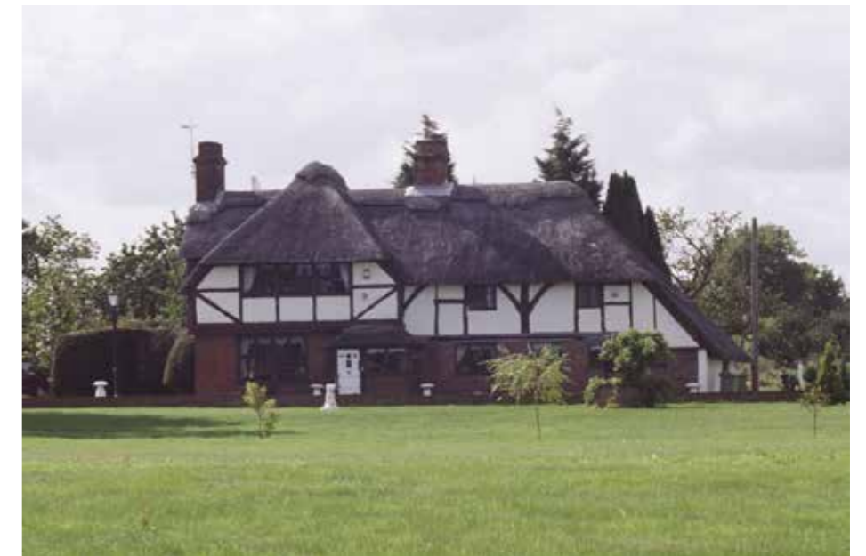
Figure 5.50 Principal east elevation of Woodstock Cottage Farmhouse
