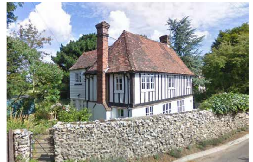
Figure 5.74 Church Cottage as viewed from Church Street to the east
