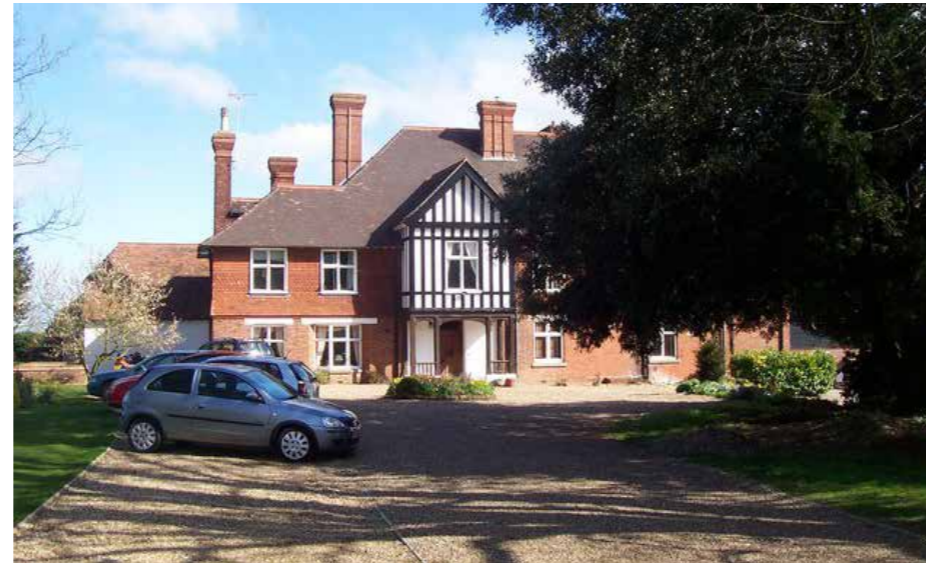
Figure 5.86 The principal south elevation of Scuttington Manor
