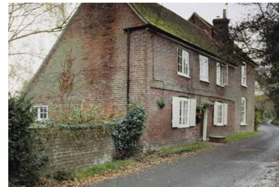
Figure 5.92 The principal south elevation of Lyndale as viewed from Ludgate Lane
