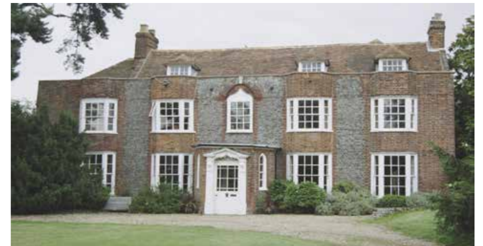
Figure 5.82 The principal west elevation of Woodstreet House
