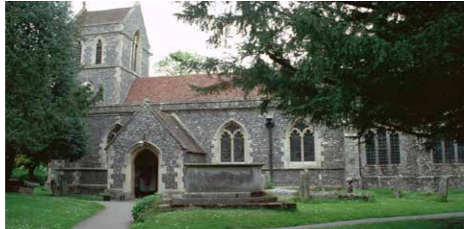
Figure 5.34 The south elevation of the Church of St John the Baptist
