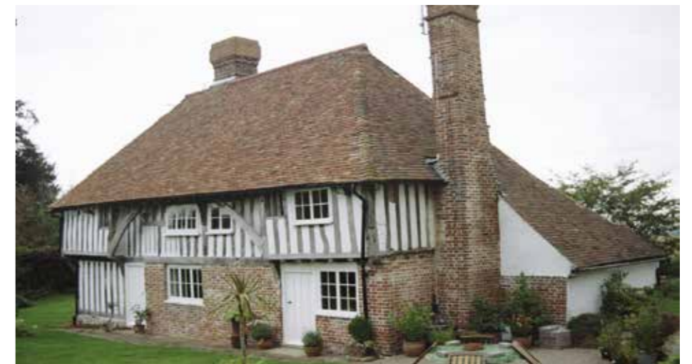
Figure 5.81 The principal south elevation of Woodstreet Cottage
