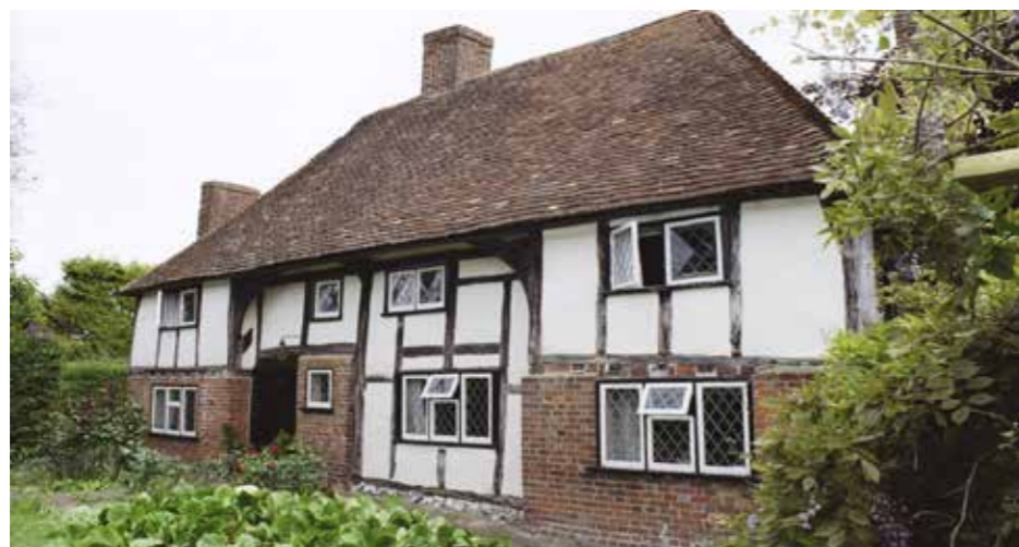
Figure 5.65 The principal east elevation of Holy Tree Lodge
