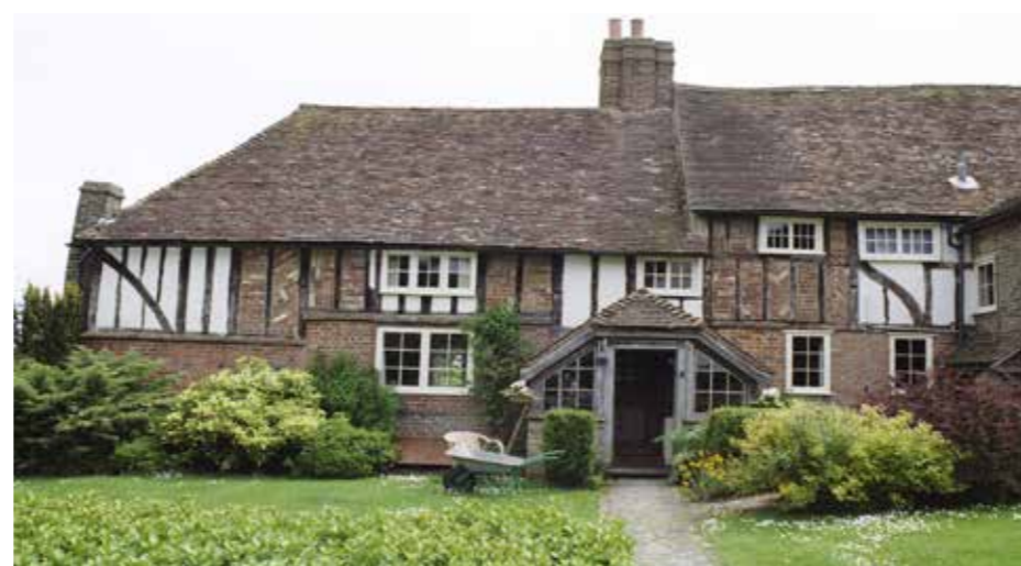
Figure 5.67 The principal west elevation of Baker Cottages
