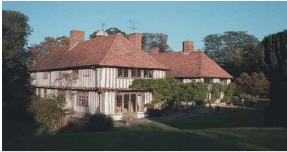
Figure 5.55 The east and rear south elevation of Milstead Manor
