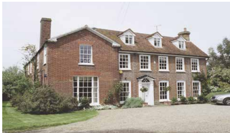
Figure 5.75 Church House as viewed from the east driveway
