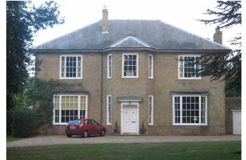
Figure 5.41 The principal west elevation of Cedar House
