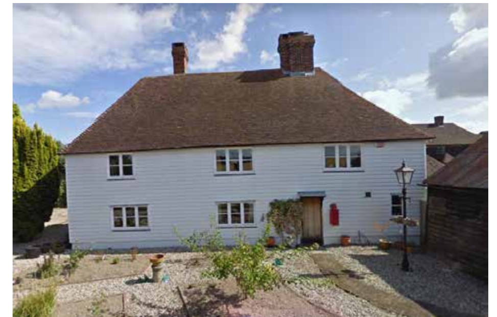
Figure 5.84 The principal south elevation of the Orchard Farmhouse
