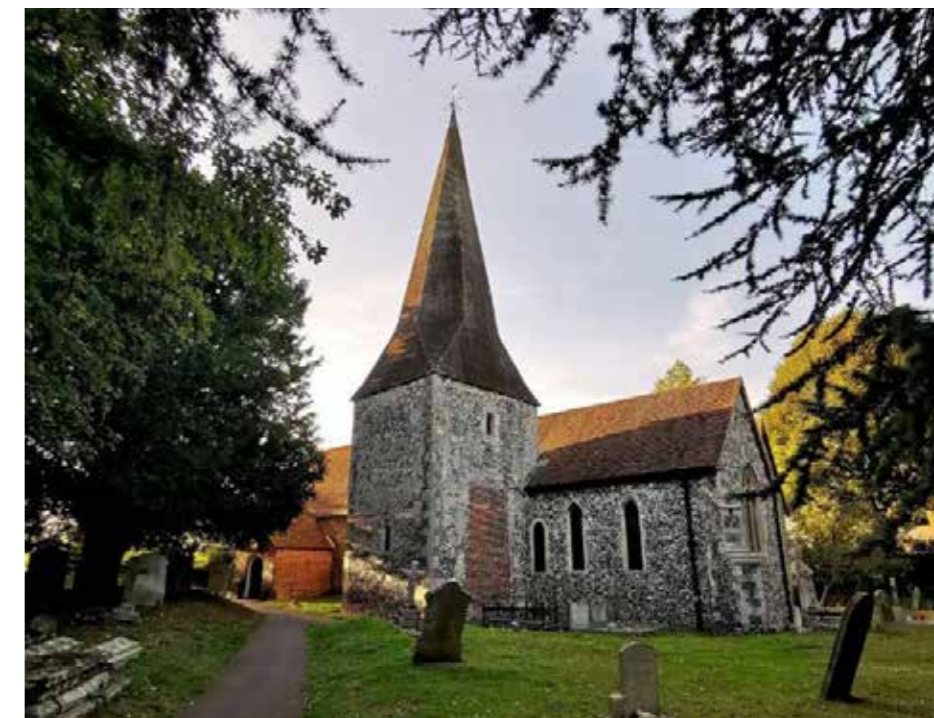
Figure 5.68 Church of St Lawrence as viewed from the southern entrance path
