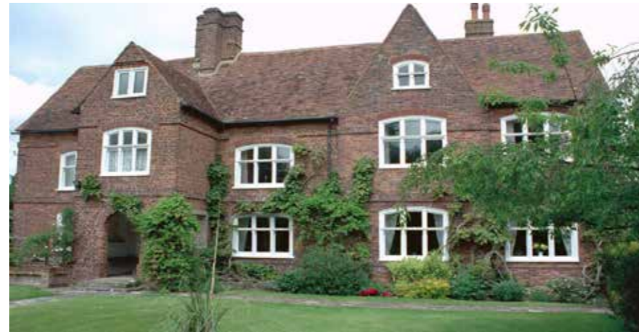
Figure 5.45 The principal south elevation of Hales House
