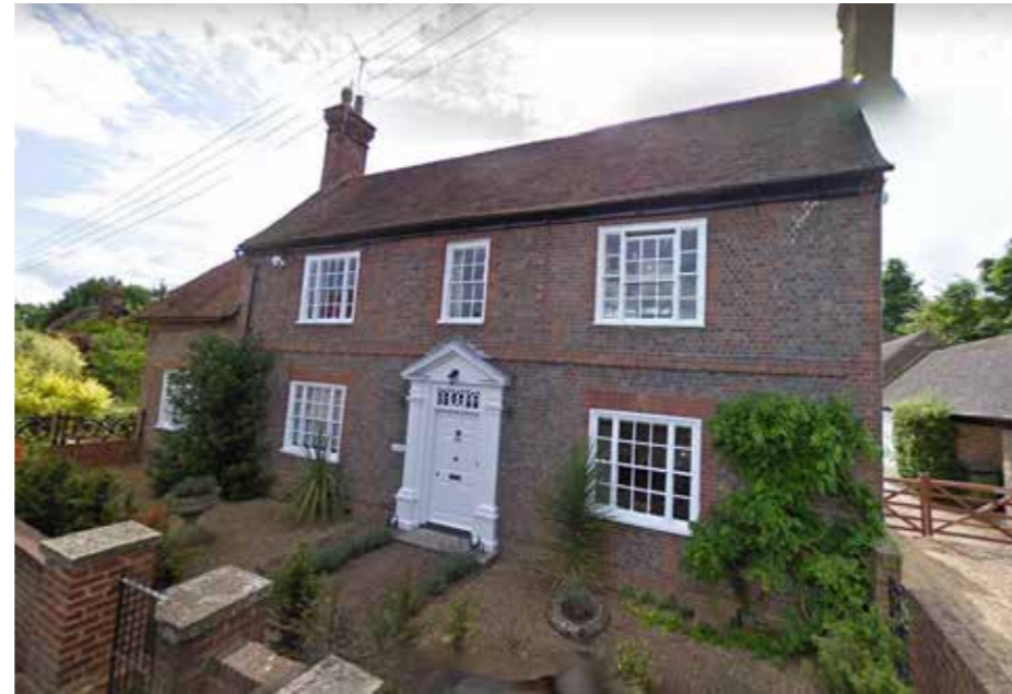
Figure 5.40 The principal north elevation of The Den
