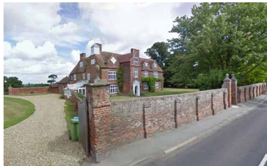
Figure 5.37 Tunstall House and its walls as viewed from Tunstall Road
