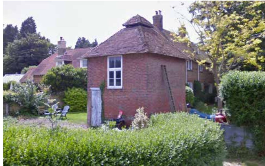
Figure 5.57 The Dovecote 50 Yard East of Milstead Manor viewed from the east
