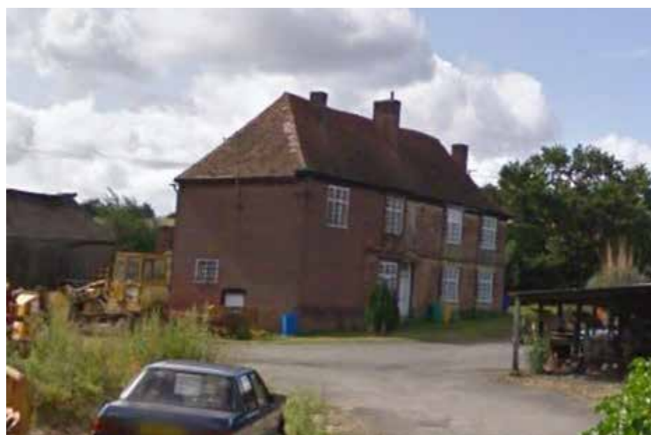
Figure 5.72 Morris Court Farmhouse as viewed from School Lane
