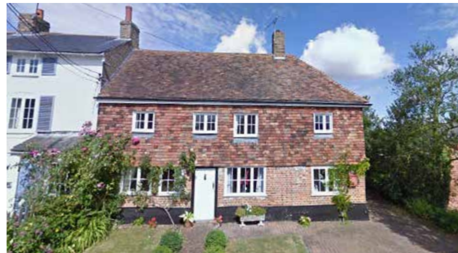
Figure 5.62 The principal east elevation of Vine Cottages
