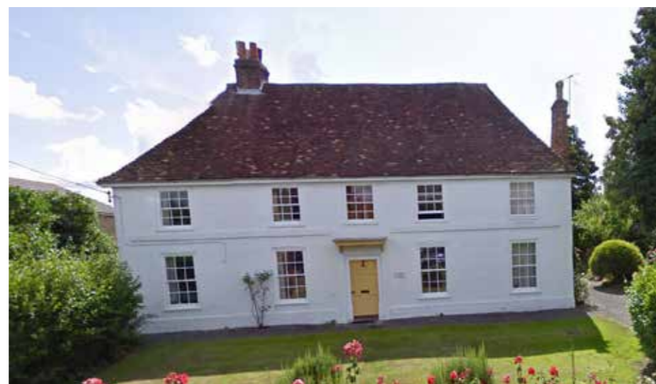
Figure 5.19 Primrose House viewed from The Street
