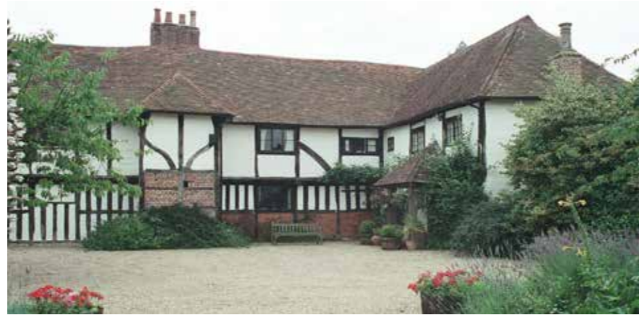
Figure 5.24 Grove End Farmhouse
