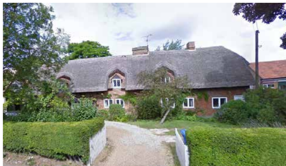
Figure 5.42 The principal south-east elevation of The Oast viewed from Tunstall Road
