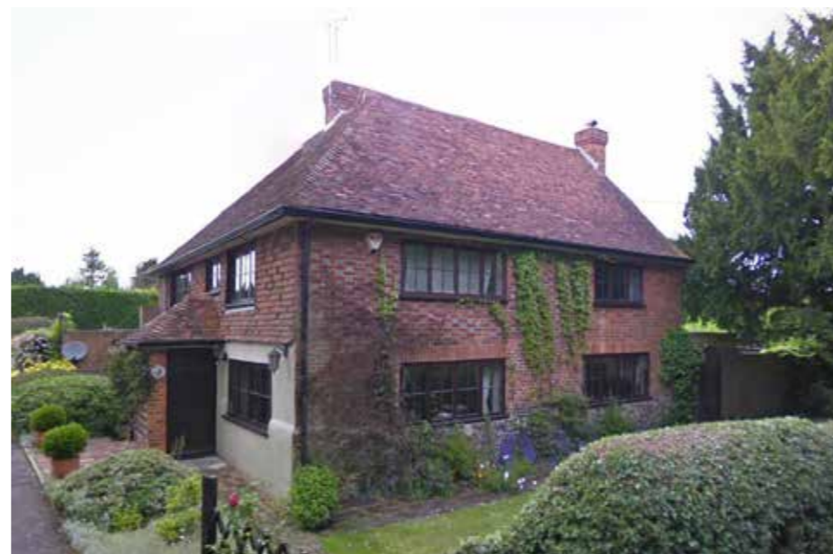
Figure 5.30 Yew Tree Cottage viewed from Hawks Hill Lane
