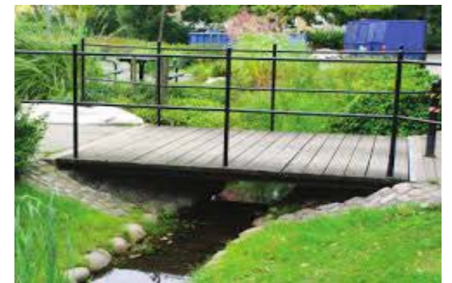
Timber bridge for connectivity
