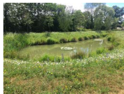
Planted attenuation basin
