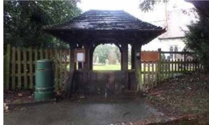
walls with brick caps
