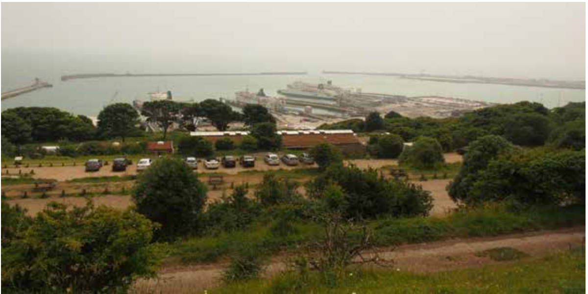
The White Cliffs of Dover Visitor Centre (with green roof) and associated car park above Dover Harbour and ferry terminal
