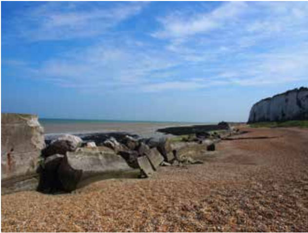
Seawall toppled by storm, Kingsdown
