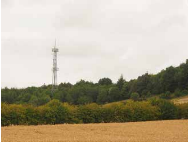
Telecommunications mast on valley side near Wye
