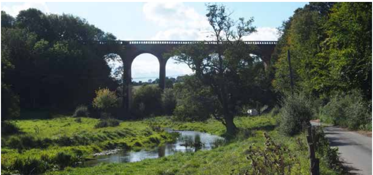
Darent Valley scene near Eynsford. The chalk slopes of the valley side can be seen between the arches of Eynsford Viaduct. In the foreground, the River Darent winds between water meadows
