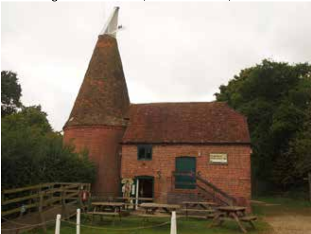
Traditional Oast House, formerly the Bough Beech Visitor Centre
