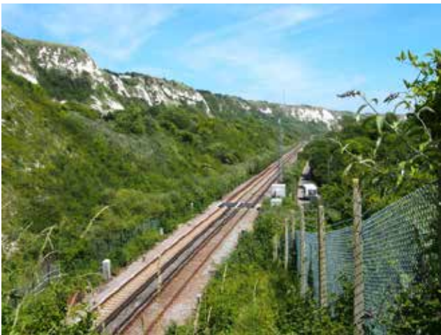
Landslips are not uncommon at The Warren, and the coastal railway line requires sea defences.
