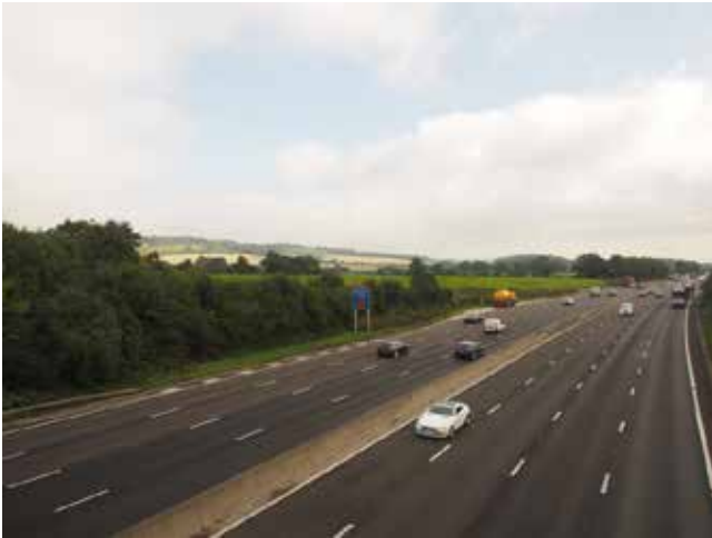
M25 running through the Darent Valley LCA near Westerham
