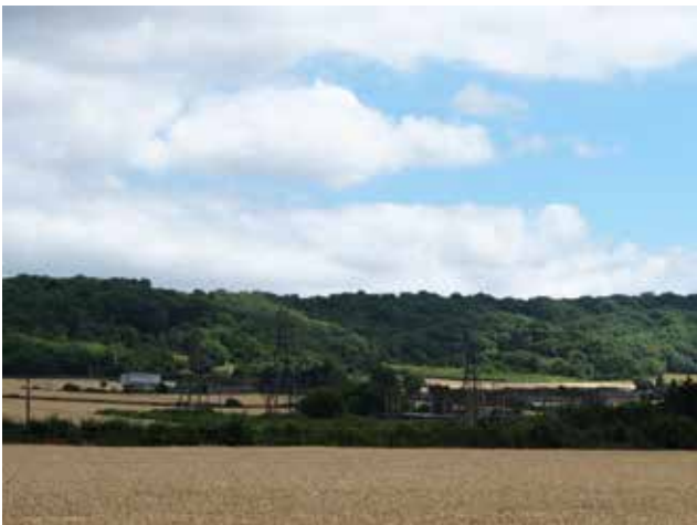
Pylons and substation near Wouldham
